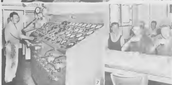
THIS CYCLONE, left, which separates dredgings from water, is the first one ever used on a commercial dredge. The idea to use this device came when the dredgers decided to use hopper barges instead of the customary floating pipelines. Dredgings, sand and coral, are loaded on the barges with this T-shaped device, right. The barges take the material out to sea to be dumped.
